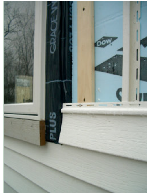
The peel-and-stick membrane air barrier on this window connects with the housewrap air barrier under the rigid-foam insulation, which is in turn under strapping and vinyl siding.
