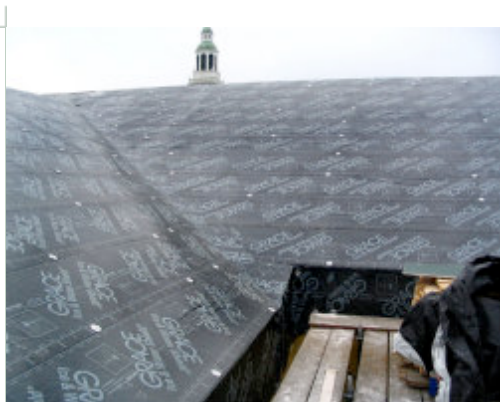
The roof air barrier for a new building at
