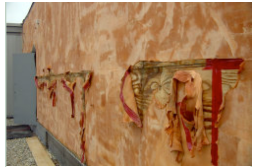
This air barrier on a Burlington, Vermont, mechanical penthouse—a spray-applied membrane over plywood sheathing with taped joints—is failing due to water infiltration at the roof-wall intersection. It was under construction and set to be covered by metal siding, which would have concealed the problem.
