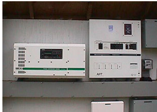
An inverter (left) and charge controller (right) are the power conditioning components of a PV system.
