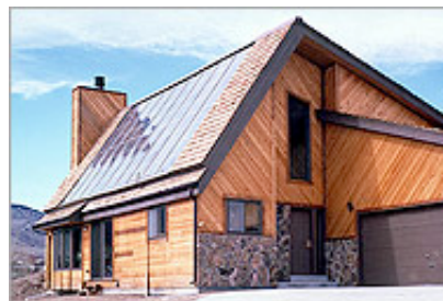
This home in Golden, Colorado uses a liquid-based solar system for space and water heating. Photo credit: Warren Gretz.
