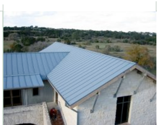
Roof overhangs, gutters, and downspouts help to prevent rainwater intrusion into buildings. Shown here is the Ladybird Johnson Wildflower Center in Austin, Texas, which also has an extensive rainwater harvesting system.
